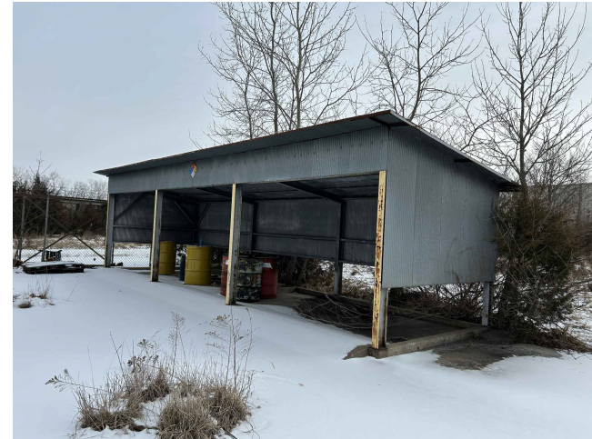
BUILDING 7 TO BE DEMOLISHED
