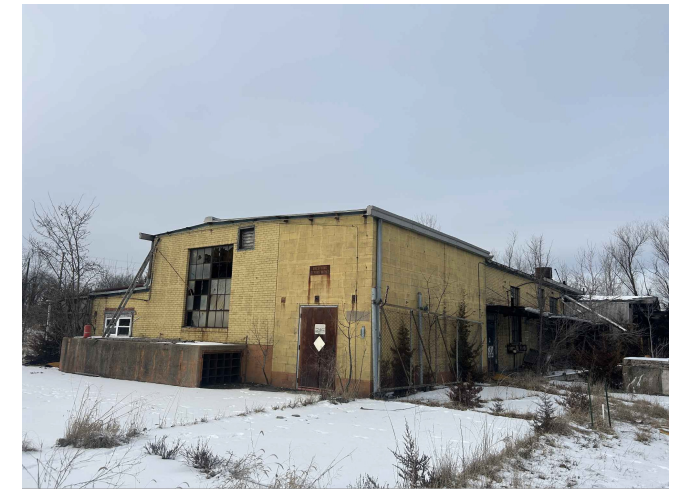
BUILDING 6 TO BE DEMOLISHED - VIEWED FROM THE SOUTHEAST
