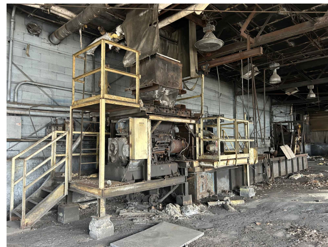
INTERIOR OF BUILDING 9 - DEFUNCT EQUIPMENT TO BE REMOVED
