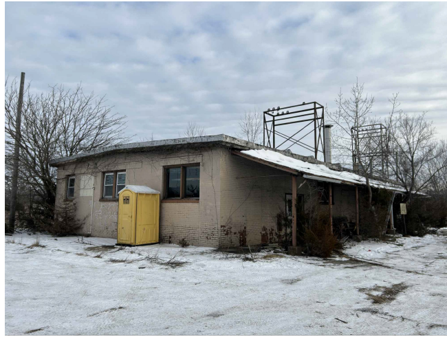
BUILDING 3 TO BE DEMOLISHED
