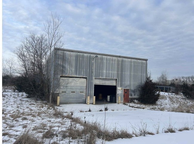
BUILDING 6 TO BE DEMOLISHED - VIEWED FROM THE WEST
