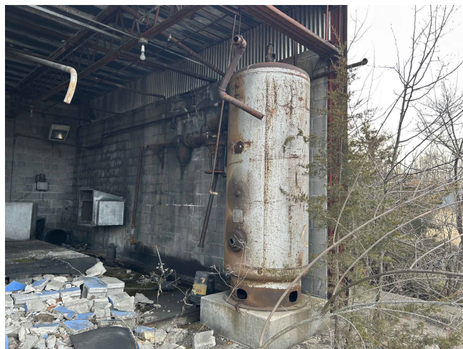
INTERIOR OF BUILDING 9 - TANK TO BE REMOVED
