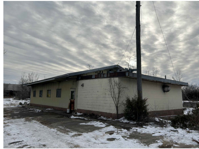
BUILDING 4 TO BE DEMOLISHED
