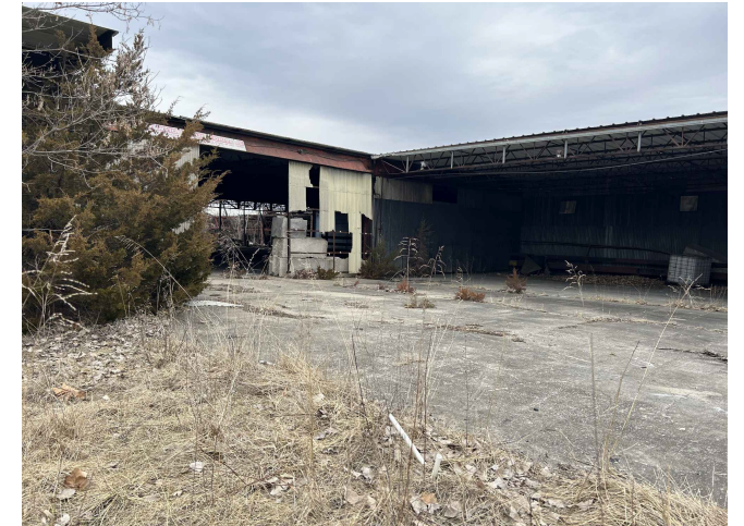
BUILDING 9 TO BE DEMOLISHED
