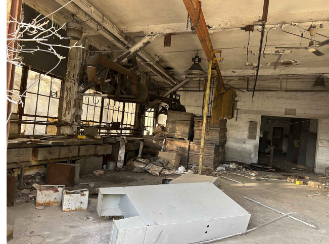
INTERIOR OF BUILDING 6 - STORED MATERIALS TO BE REMOVED
