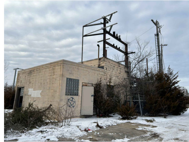
BUILDING 5 TO BE DEMOLISHED
