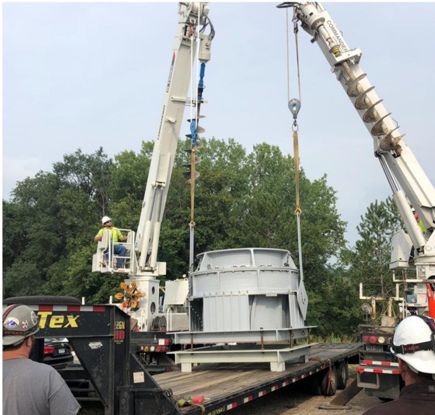
Off-loading turbine on dam
