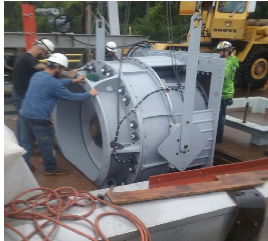
Installation of turbine in pit
